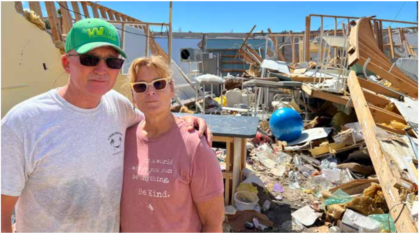
Teresa and Dave Karaffa inside their Englewood business, the Lemon Bay Soap Company, which was destroyed by Hurricane Ian. The roof of the business came completely off, with nothing overhead but blue sky. Photo credit: Zac Anderson, Sarasota Herald-Tribune
